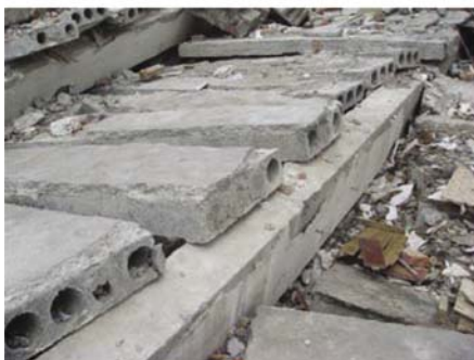
Fig. 14 Poor connections between precast RC floor slabs and tie-beam
