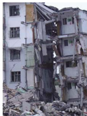
Fig. 14 Poor connections between precast RC floor slabs and tie-beam
