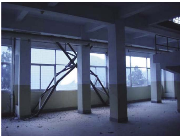
Fig. 4 Buckling brace between columns of an industrial building in Yingxiu Town (VII/XI) of Anxian County (VII/VIII)
