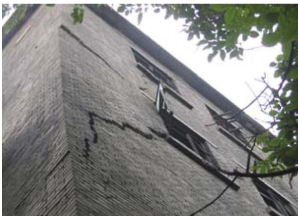
Fig. 21 Rotation at upper corner of a masonry building (VII/VIII)
