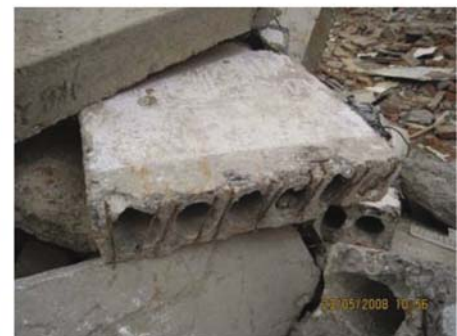
Fig. 14 Poor connections between precast RC floor slabs and tie-beam
