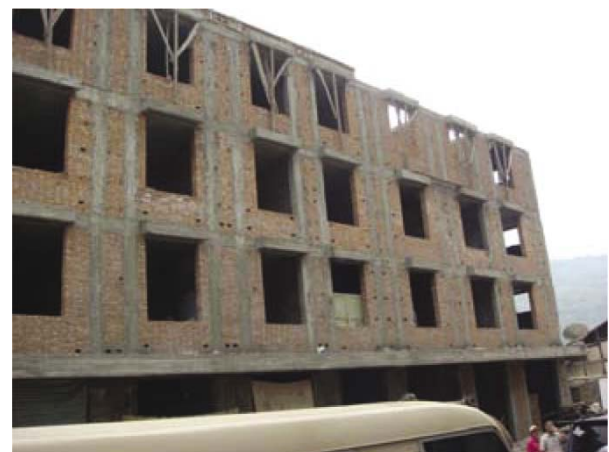
Fig. 6 Confined masonry building at the rear of that in Fig. 5
