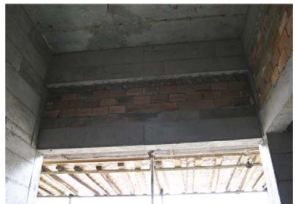
Fig. 11 Twin coupling beam of a frame-shear wall structure in Chengdu City (VII/(VI-VII))
