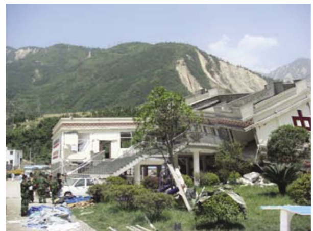
Fig. 2 Collapsed school building (right) in Yingxiu Town (VII/XI)
